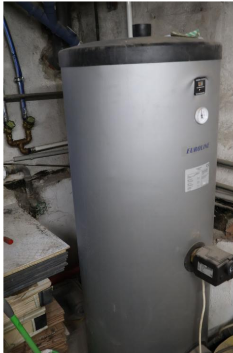
E-Warmwasserboiler
